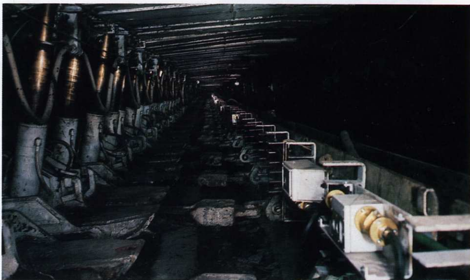
F.110's installed face.
