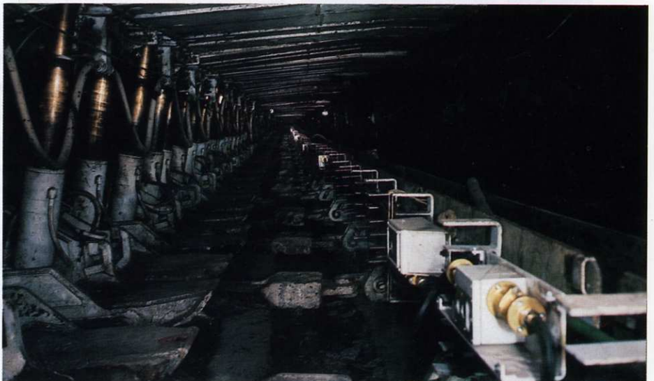
F.110's installed face.
